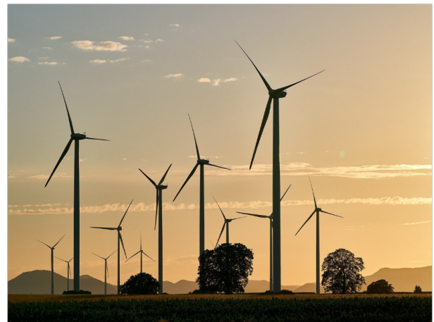
Optimization and maintenance of wind turbines
