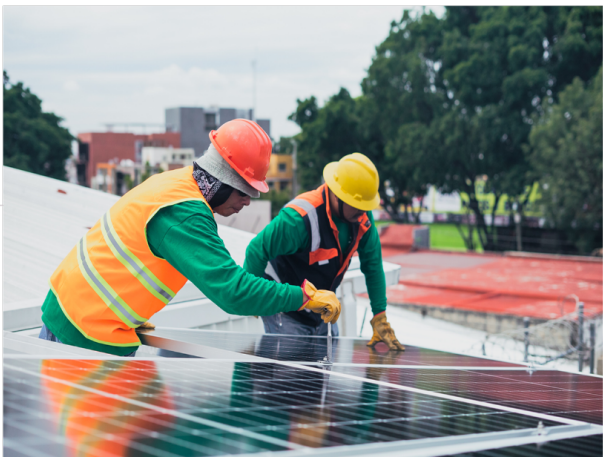
Installation and maintenance of photovoltaic panels
